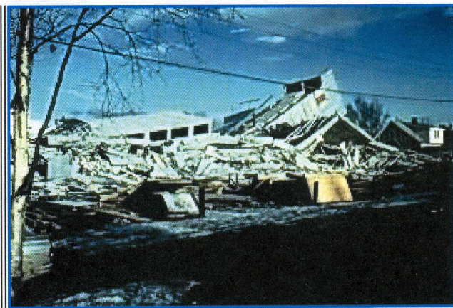
The six-story Four Seasons apartment building in Anchorage was completely destroyed. It was unoccupied at the time of the earthquake.
